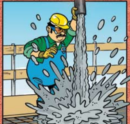
AVOID SEGREGATION. DO NOT ALLOW CONCRETE TO FALL FROM TOO GREAT A HEIGHT.
