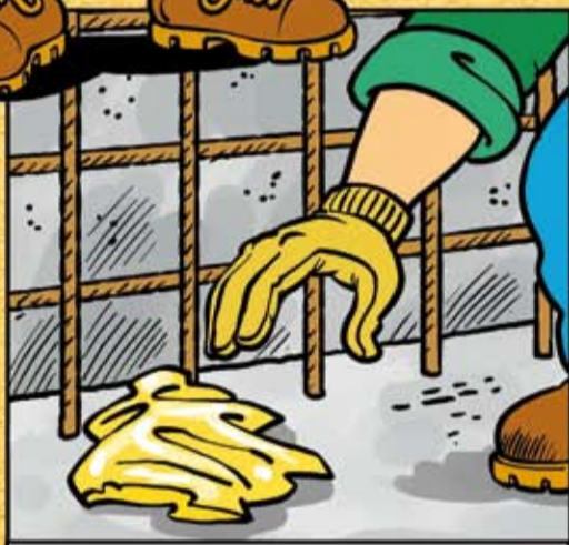
REMOVE ANY LITTER FROM THE FORMWORK.
