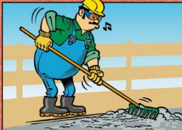
IF IT IS NECESSARY TO MOVE CONCRETE, USE A SHOVEL OR A RAKE, NOT THE POKER VIBRATOR.
